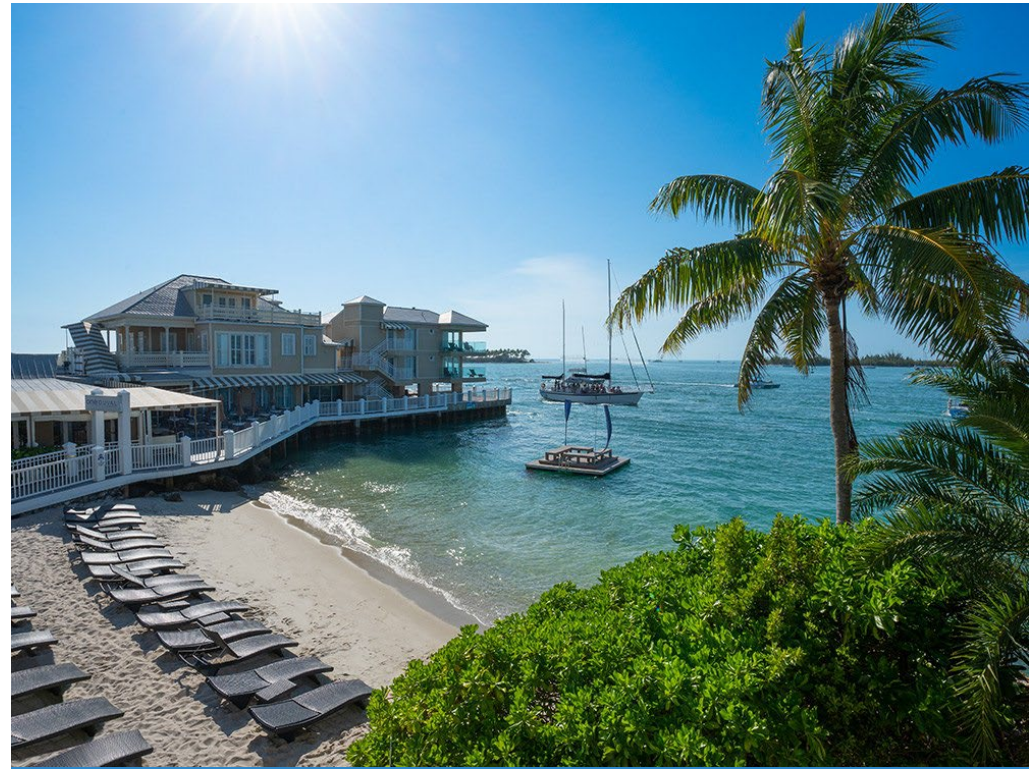
Pier House Resort and Spa
